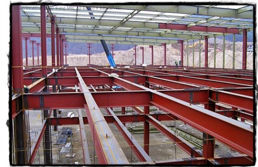
Iron structure building
