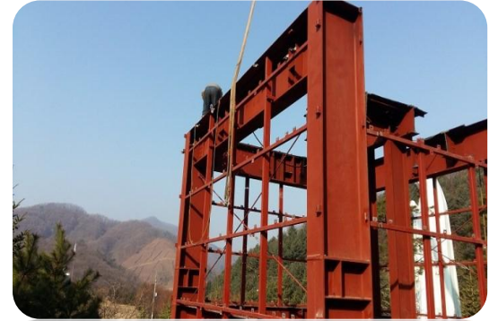
Iron structure building
