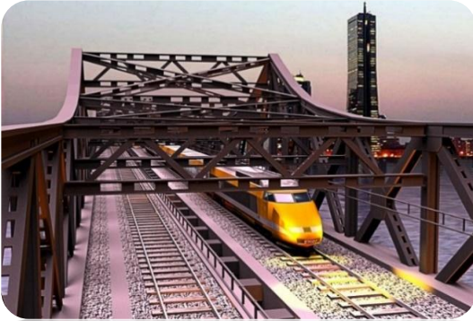
Steel structure bridge
