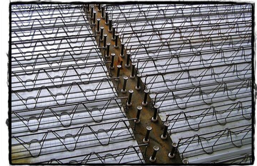
Iron structure building
