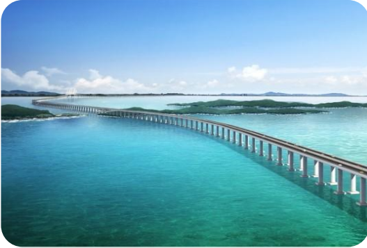
Steel structure bridge
