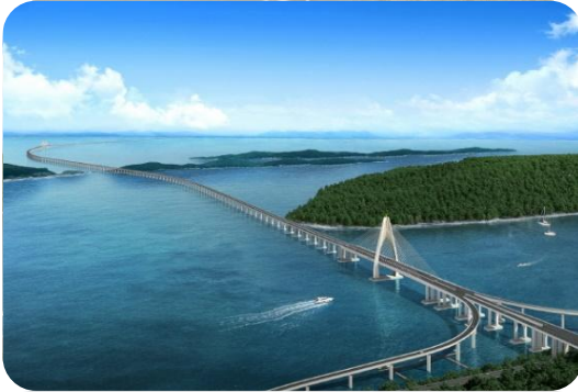
Steel structure bridge
