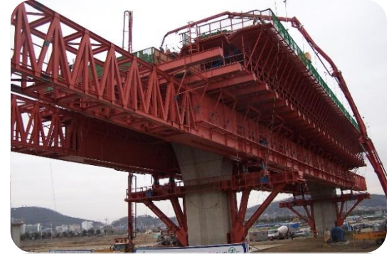
Iron structure building
