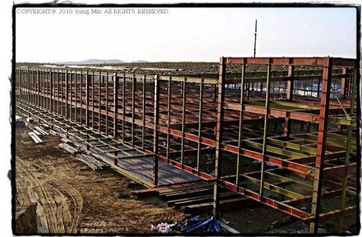
Iron structure building
